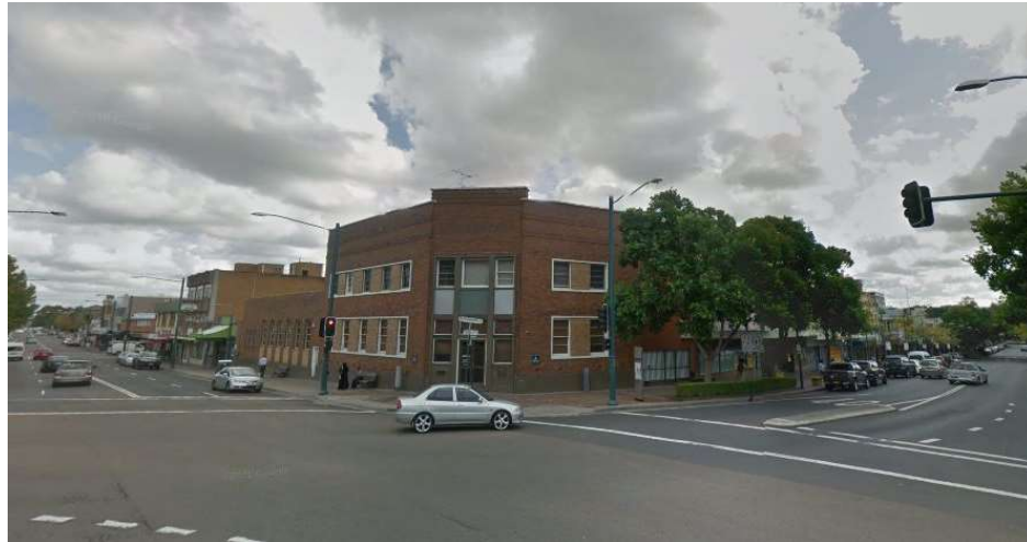
Figure 22 - View of the Commercial Building from the general area of the subject site. (Source: Google Streetview)
